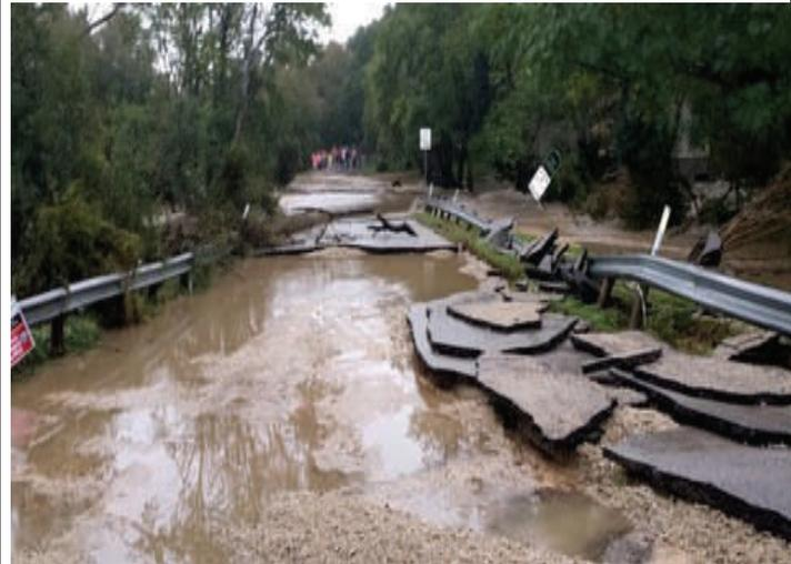
**10.31.13 Flood waters stripped the asphalt surface from the Twin Creeks bridge road bed over Onion Creek**
