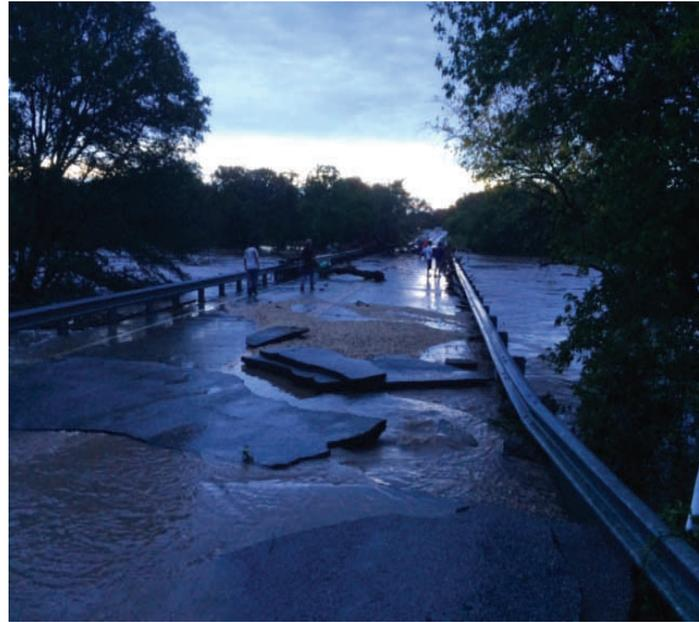
**10.31.13- Note that waters of Onion Creek and Bear Creek (above) rose over the road bed on the Twin Creeks Rd. bridge. The bridge is normally 20 ft. above the creeks. On both sides of the guard rails the receding creek is still just below the bridge decking.**
